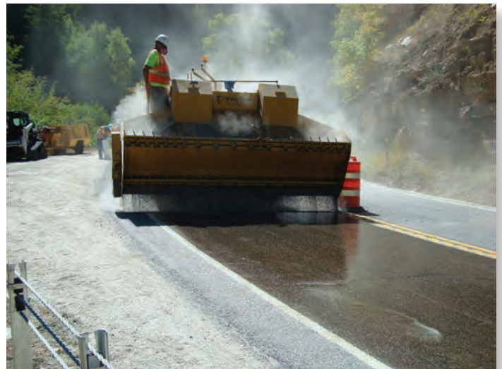
Mechanical installation of HFST (Image: David Merritt)
