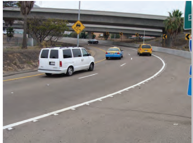
Sepulveda ramp HFST installation (Image: California Department of Transportation)
