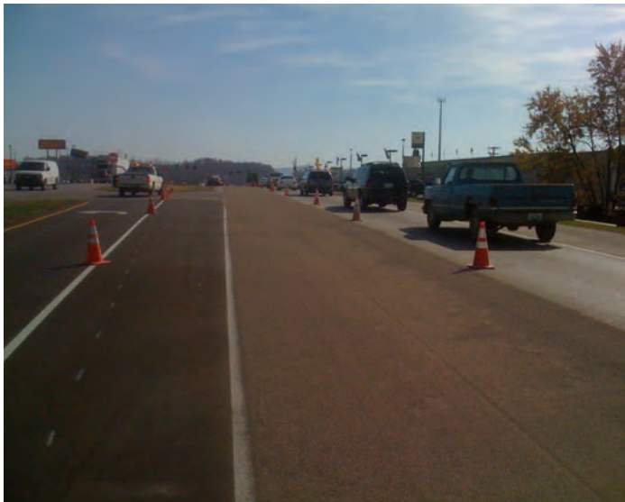
Overview of the US 25 - KY 1629 intersection site (Image: Kentucky Transportation Cabinet)
