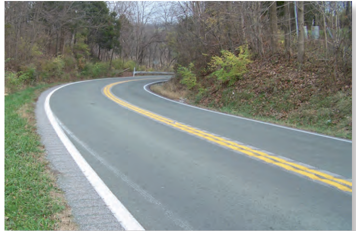
Overview of the KY-22 site at milepost 4.36-4.44 (Image: Kentucky Transportation Cabinet)
