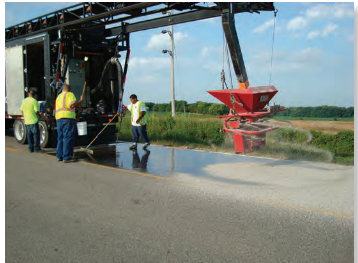
Different mechanical means can be used to install HFST (Image: David Merritt)
