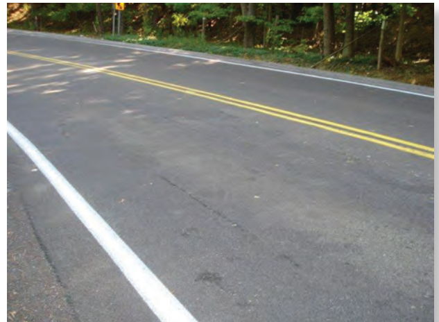
WV20, Between Princeton and Athens (Image: West Virginia Department of Transportation)
