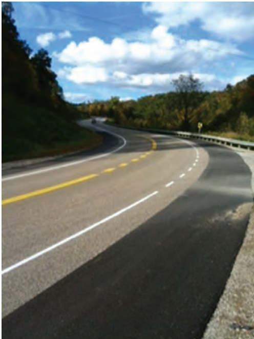
WV14, north of Elizabeth (Image: West Virginia Department of Transportation)
