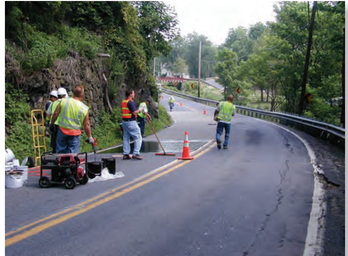
Binder materials can be applied mechanically or by hand, as shown (Image: Pennsylvania DOT)
