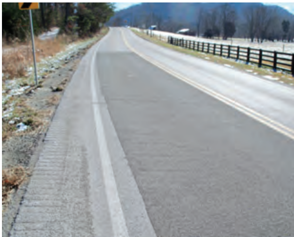
Overview of the KY-21 site at milepost 11.3-13.6 (Image: Kentucky Transportation Cabinet)
