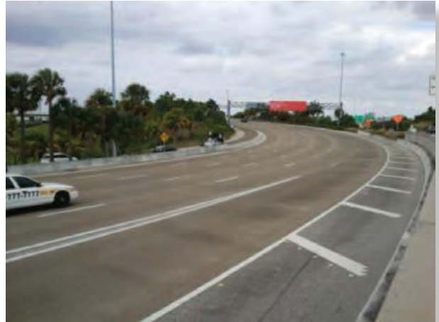
I-595 ramp to the Ft. Lauderdale airport HFST installation (Image: Florida Department of Transportation)
